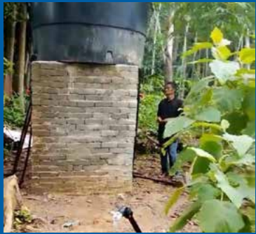
Well, water tank & hose
